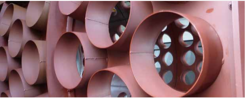
Protection against wrapping by pipe sleeves
