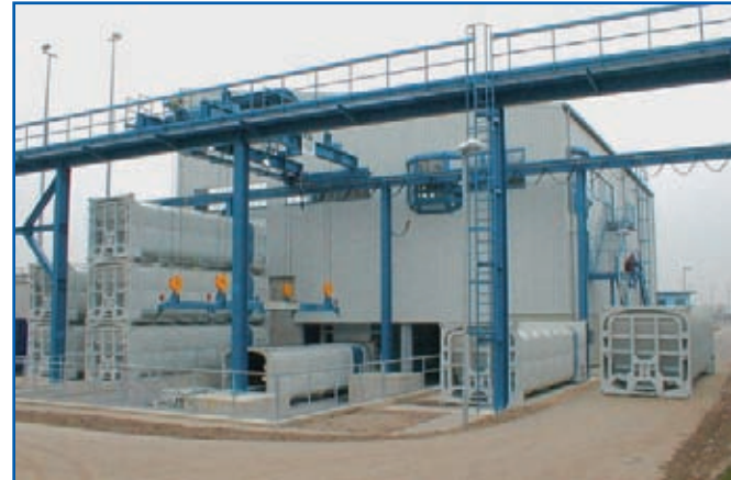
Waste transfer station
